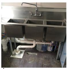
This sink has a "broken drain" which provides an air gap to prevent back flow.
